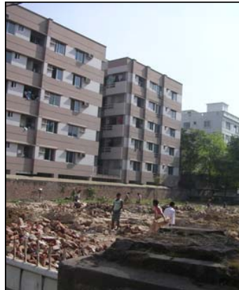
Fig. 6 Demolishing & Rebuilding by Informal Sector
